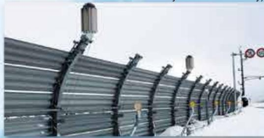
Road direction flash lamp powered by wind even at low velocities (Japan Parts Center Co.)
